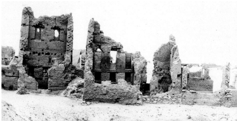
Figure 11. Multi-storeyed houses at Karanis. 72
