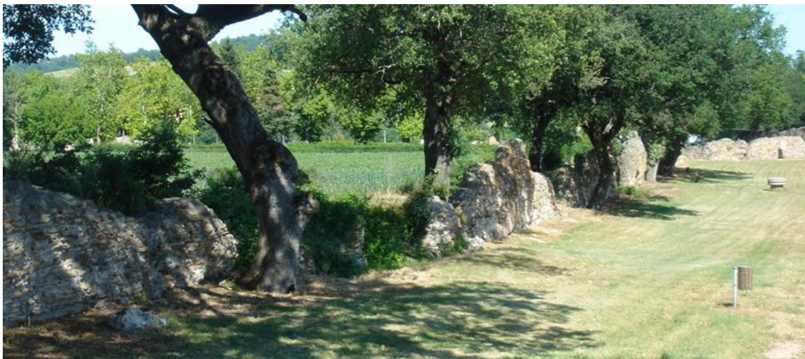
Figure 3: internal façade of city walls of Urbs Salvia, northern perimeter. © Isobel Pinder
