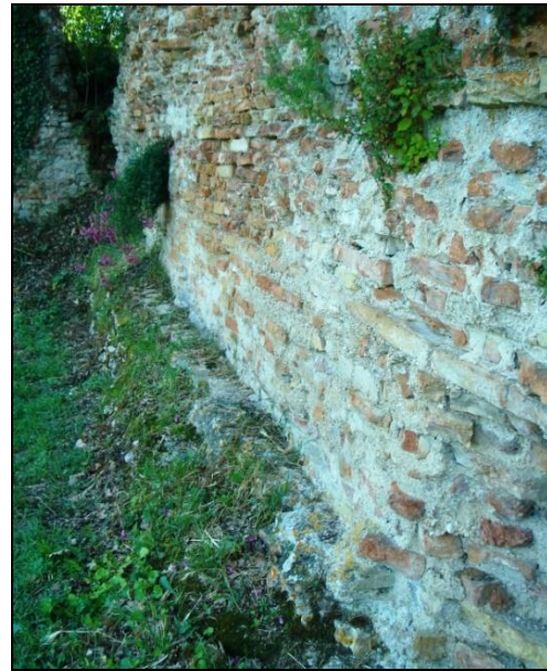
Figure 5: external wall section showing foundation plinth, northeast corner of circuit. © Isobel Pinder
