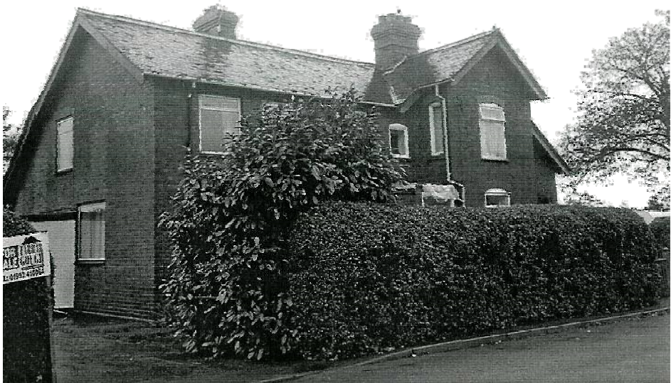
Figure 1. Lilleshall Company Hospital, Albion Street (SJ703111) South and West Aspect
